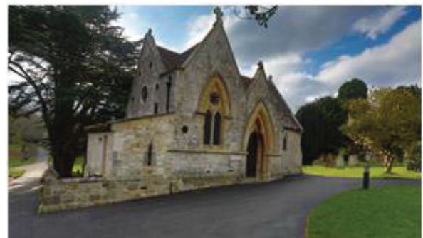
Northwood Cemetery Chapels 2018, restoration
