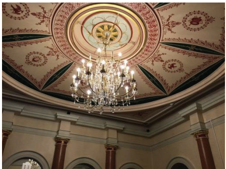
Northwood House, 2017, conservation
